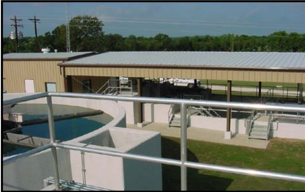
2.0 MGD WATER TREATMENT PLANT
