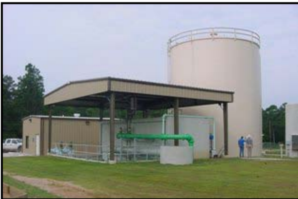
1.0 MGD FILTER BUILDING
