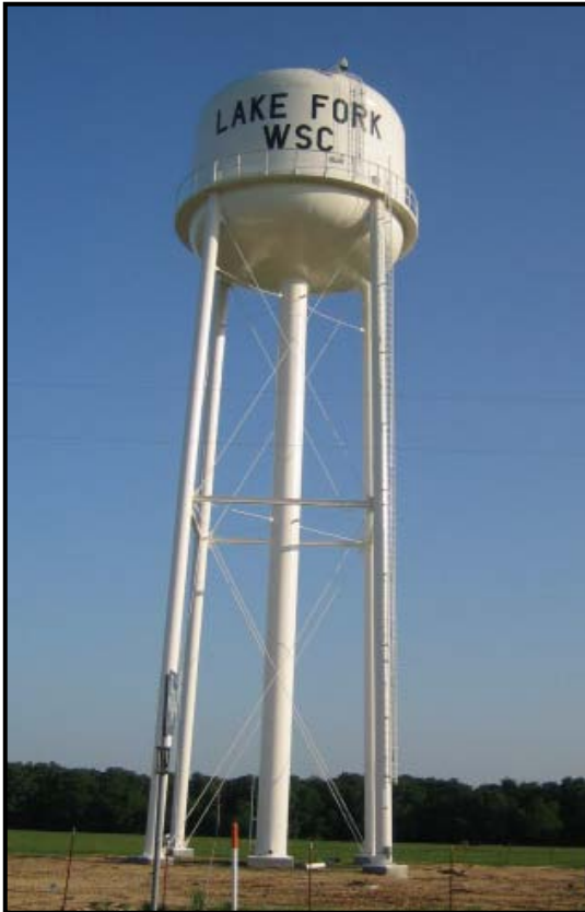
150,000 GALLON ELEVATED TANK
