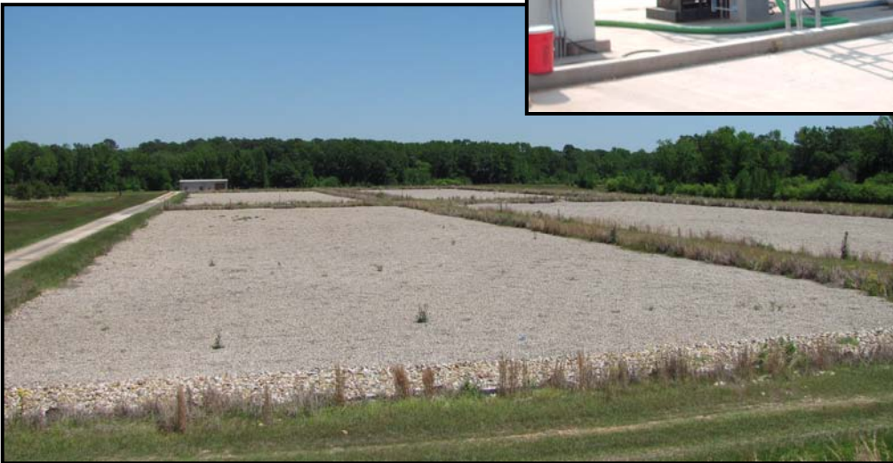
SUBSURFACE FLOW ROCK FILTER TREATMENT
