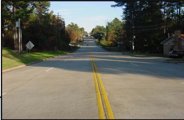
HOLLYBROOK DRIVE UNREINFORCED CONCRETE
