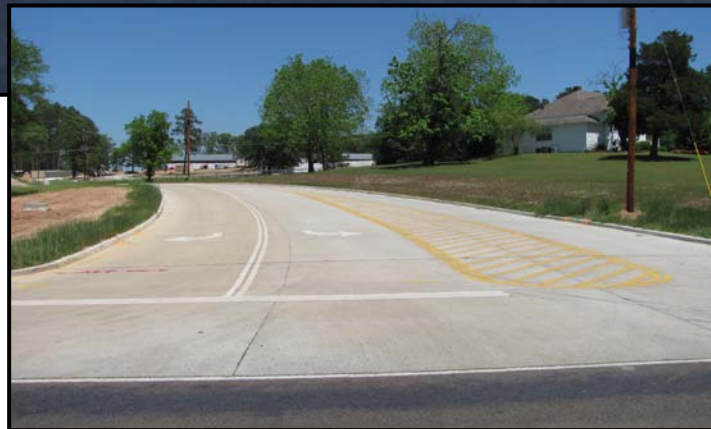
TEX HATLEY BLVD. REINFORCED CONCRETE
